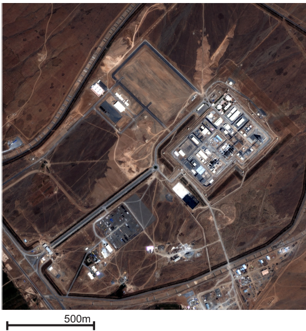
Figure 5. QUICKBIRD image of the Arak Facility, 12 June 2004 - pre-processed, original image provided by Digital Globe
