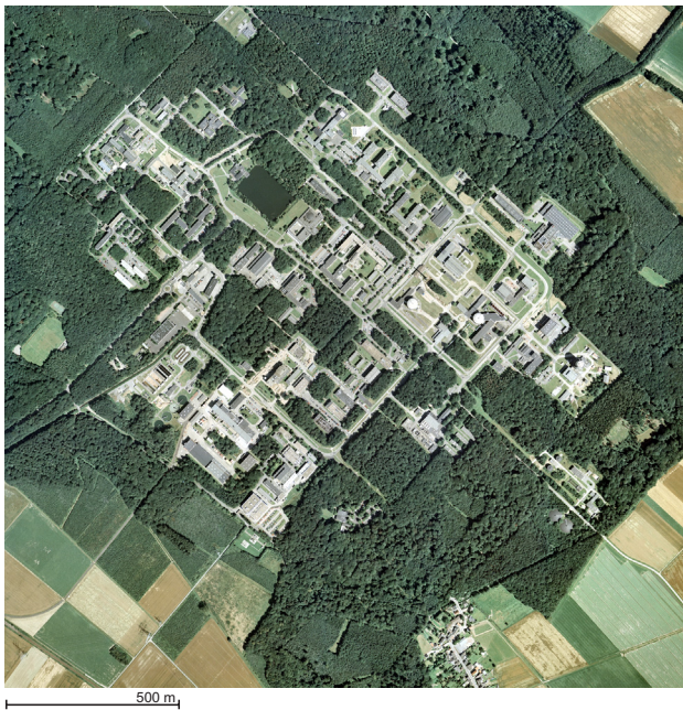
Figure 3. Research Center Jülich, September 1998
